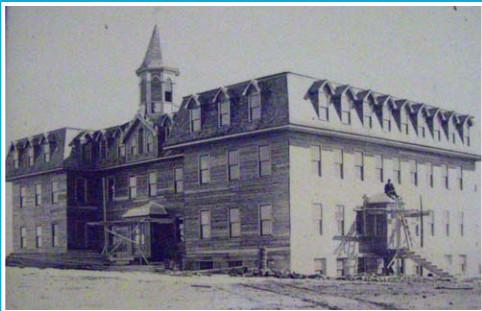
The construction of St. Mary's Hospital, Trochu
